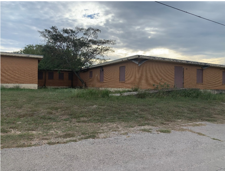
Former Nursing Home Exterior View from W. Grogan St. (Pictured former ADA compliant ramp and connecting hall from main meeting area to housing wards.)
