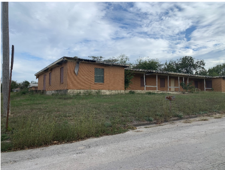
Former Nursing Home Exterior View from corner of W. Grogan St. and S. Price St.
