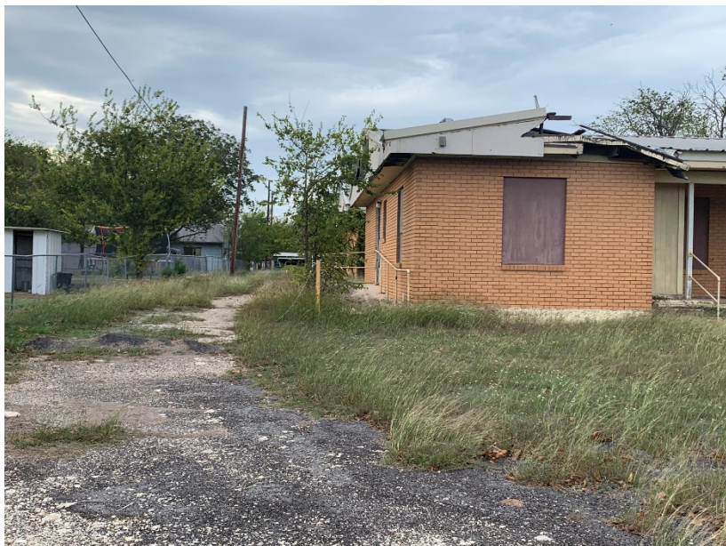
Former Nursing Home Exterior View from S. Stidham St. (Pictured backside of property with gravel alleyway.)
