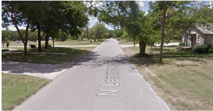
Figure 8A. Good condition.
