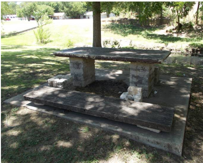
Figure 10N: Damaged Picnic Table
